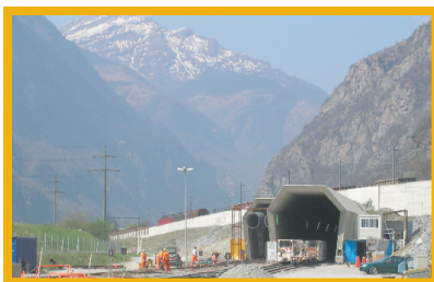
GBT entry point at Bodio.
