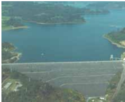
Portomouros hydroelectric dam.
