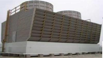
Water cooling tower for the blast furnace
